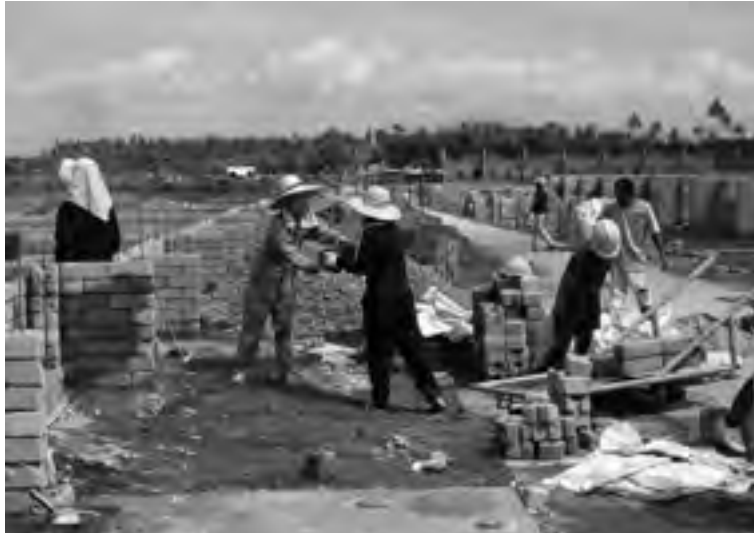
SUAC Habitat members at the build site. Caluan, Laguna, Philippines March 2011
